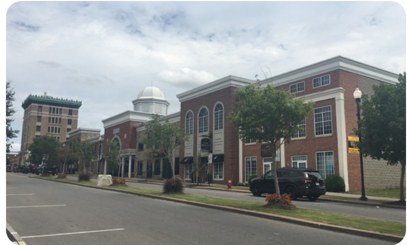
Infill development at Ulrich City Center - 80 Main Street
